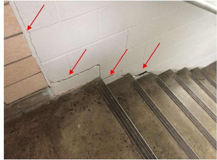
Structural movement and cracking
